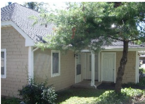
Renovated Family Housing Units – Prospect Ridge
